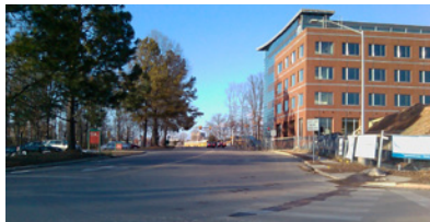
Existing George Mason Boulevard
