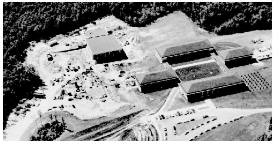
The original four buildings, the library and Lecture Hall under construction.
