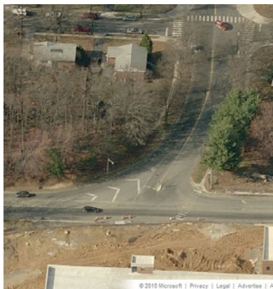
University Drive prior to construction
