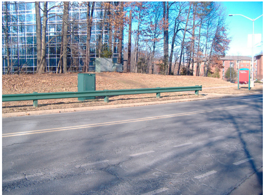
Existing guardrail used to deter jaywalking
