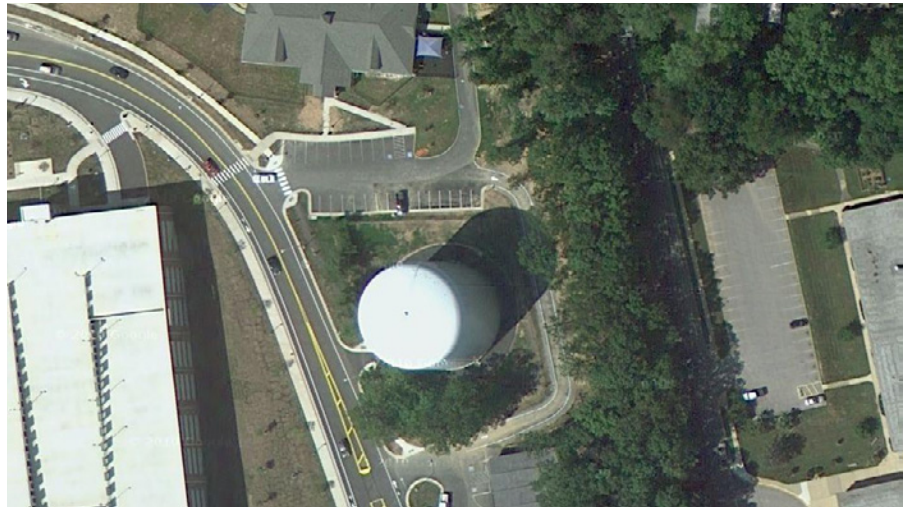
Aerial photo after construction
