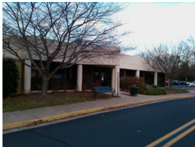
Existing parking and transportation services building
