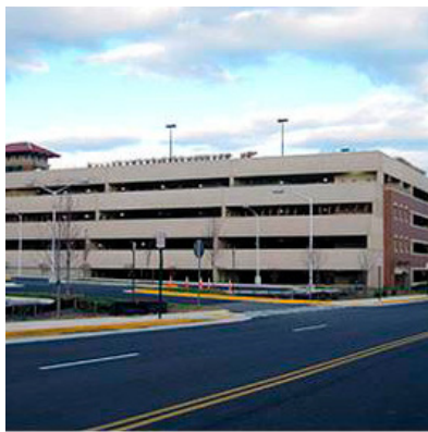
Existing VRE garage
