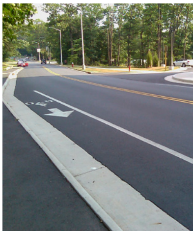
Previous end of bike lane
