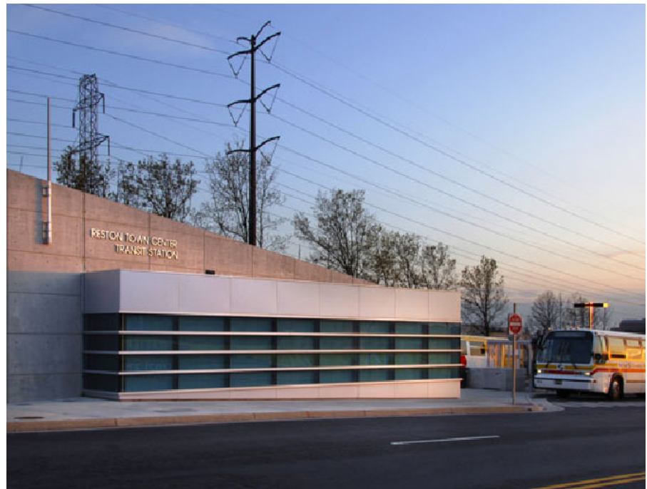
Example transit center (photo courtesy of Noritake Associates)
