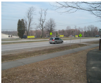
Existing crosswalk before lighting
