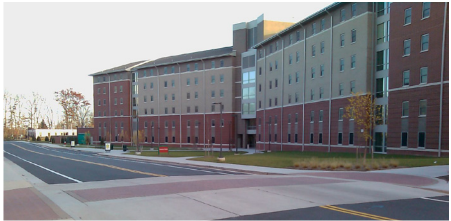
Example of a raised crosswalk near Hampton Roads
